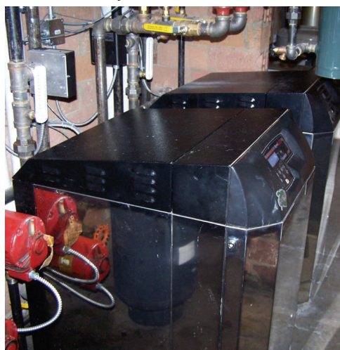
New high efficiency boiler installed at rest home
